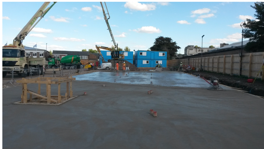
Pouring concrete foundations .
